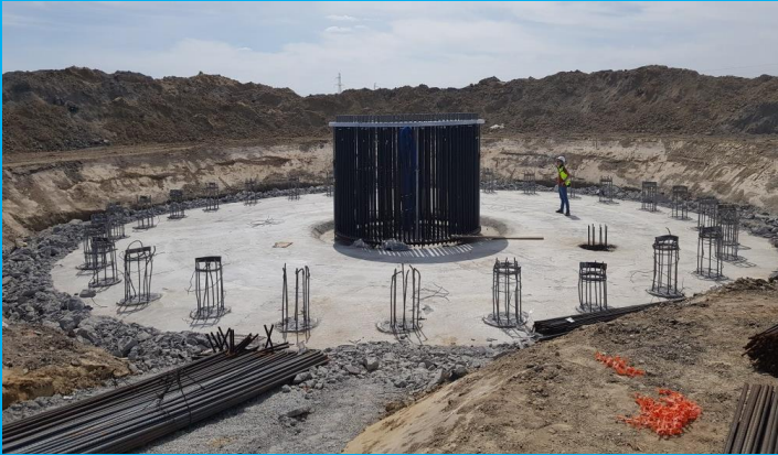
Construction of foundations for a wind turbine in Miłosław
