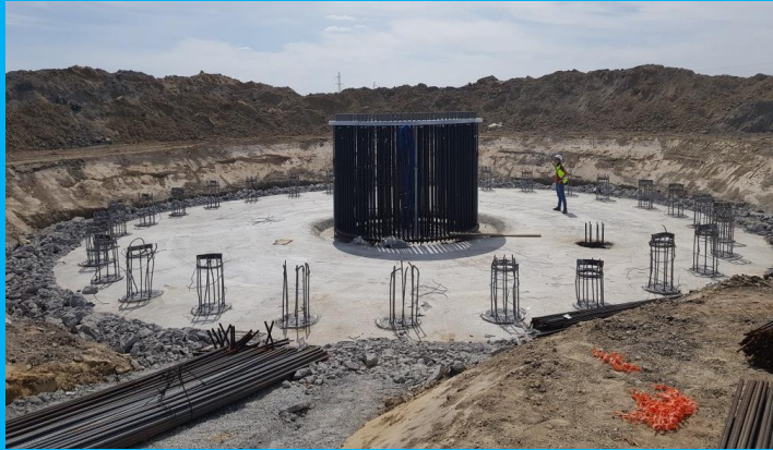
Construction of foundations for a wind turbine in Miłostów
